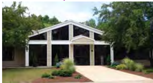
Site at 91 Northwest Drive, Plainville
